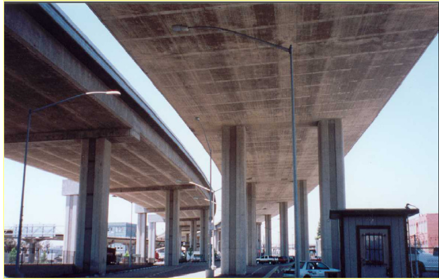
Fig. 2.1 Partial view of rebuilt I-880 viaduct
