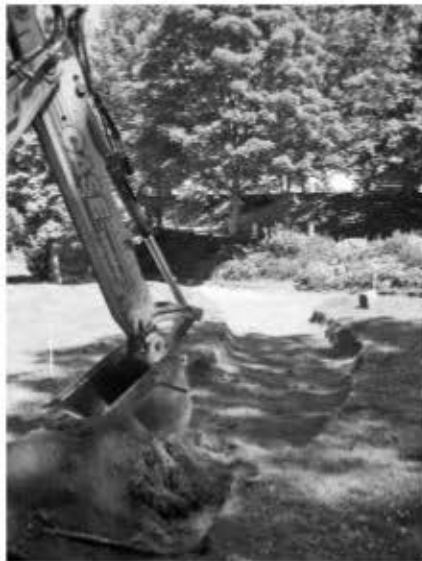
A backhoe digs out topsoil for the eight-foot-wide carriage path, which will be covered with a special stone material that was used to construct Erie Canal towpaths in the 1820s.
