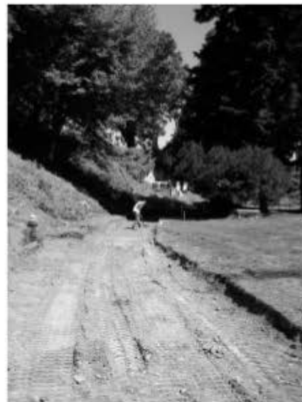
A worker rakes the excavated carriage path to level the ground before the hard surface is laid.
