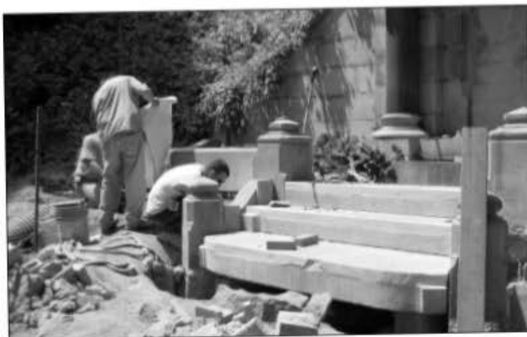
The stone steps and forecourt walls had to be completely reassembled and reset into their original positions, because the entire area in front of the Rau mausoleum had collapsed.
