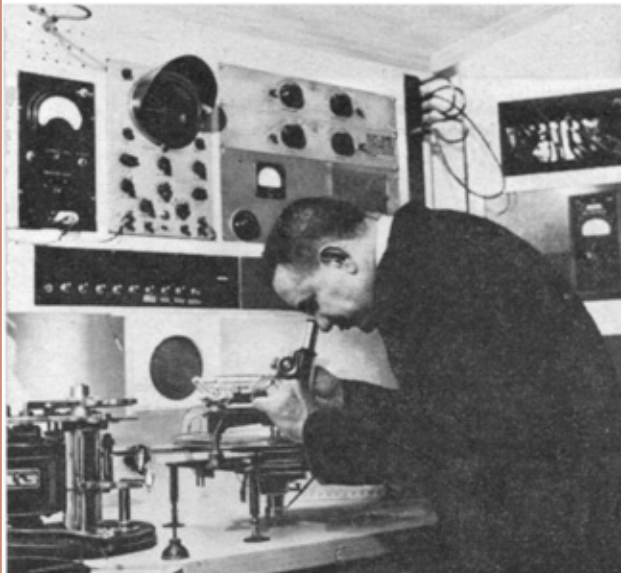
Scott uses microscope to see that grooves are cut correctly on test record made in his home studio
